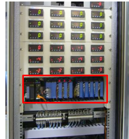
PLC and digital panel-meters for Interlock of NC magnet PS
