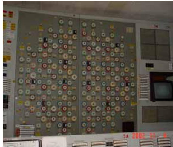
Fig. 11 Control rod position panel of 1st block
