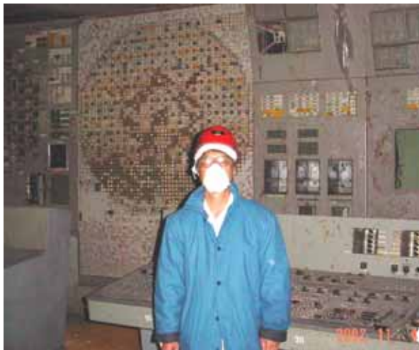
Fig. 10 Control room of 4th block. October 2002.
