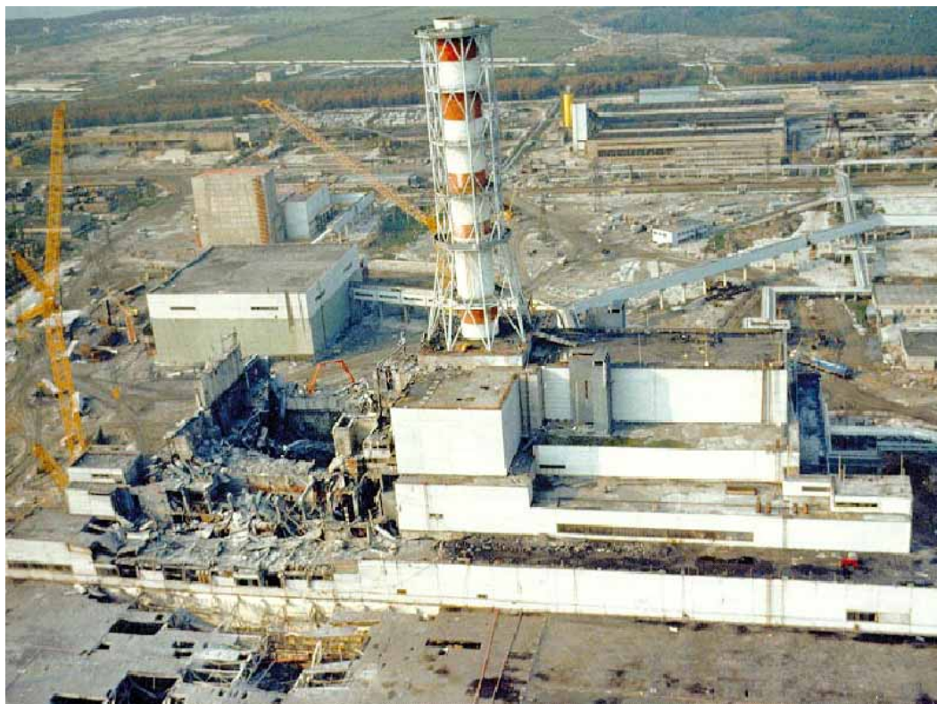
Figure 2 - Destroyed ChNPP Unit 4
