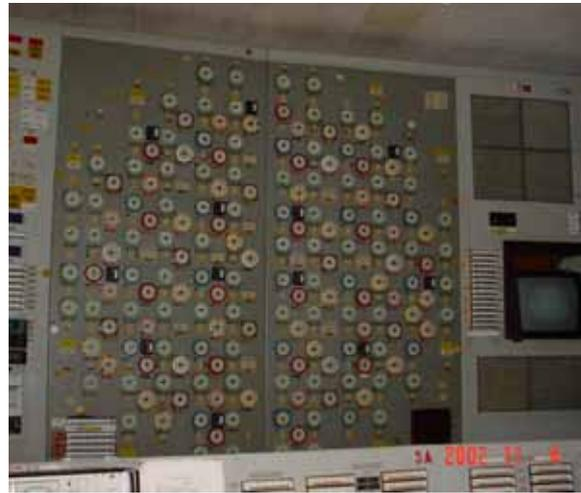
Fig. 11 Control rod position panel of 1st block
