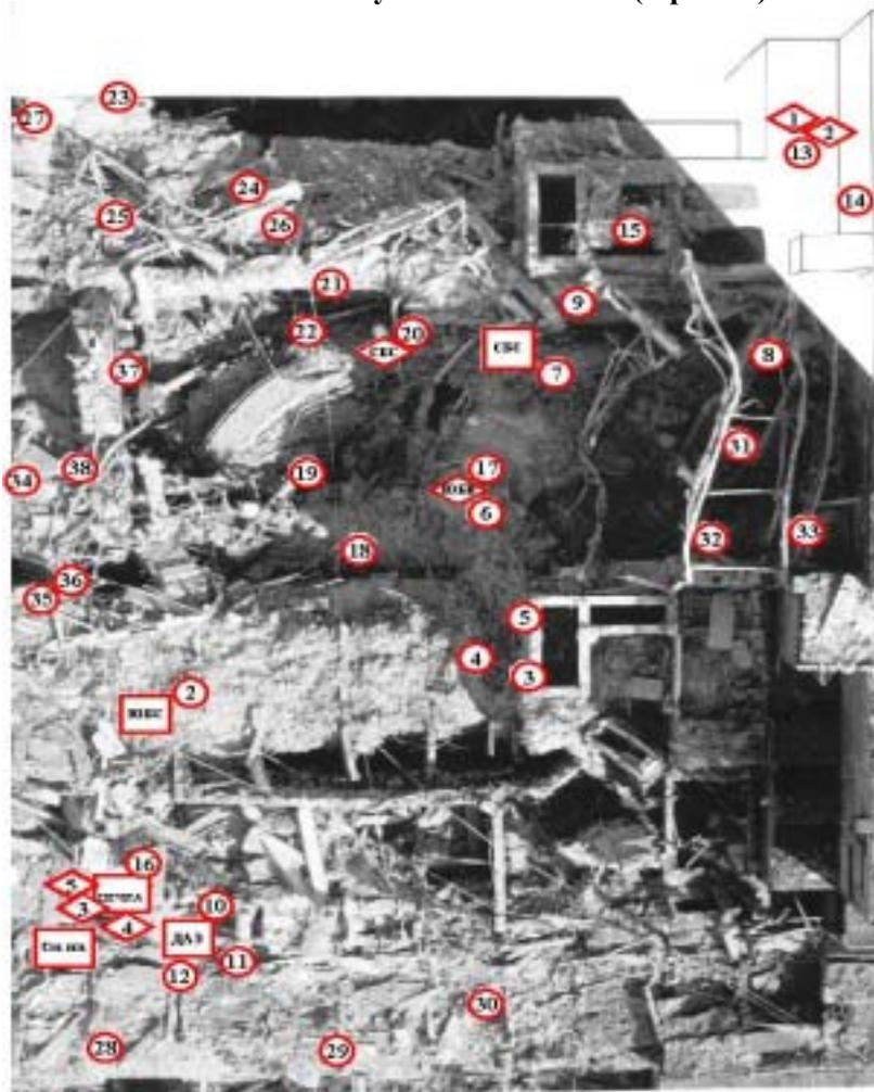
**Photo 2. The view to the Central hall of the Unit-4 reactor(side view). The points of the fuel sampling for the following investigations were marked by circles.**
