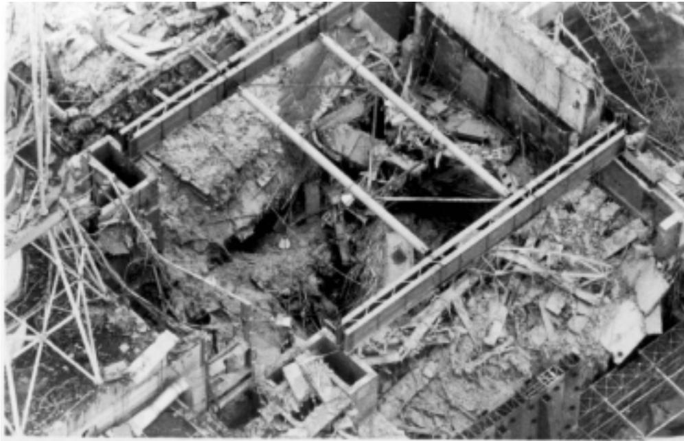
**Photo 1. The destroyed Unit-4 reactor (top view).**
