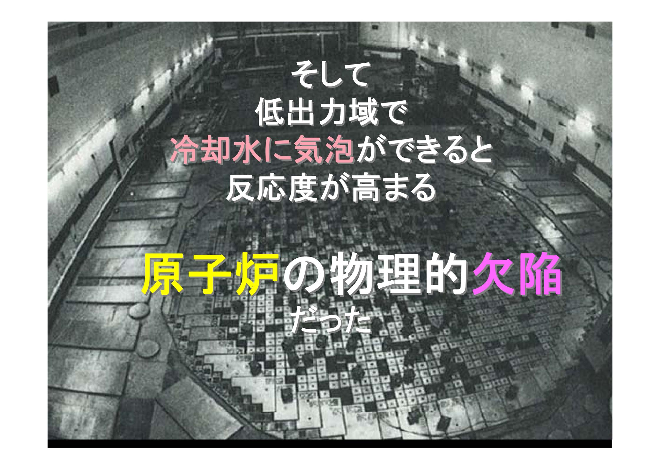
An aerial, top-down view of a nuclear reactor core. The core is a large, circular structure with a complex internal layout of fuel elements and support structures. The image is in grayscale, with some highlights from overhead lighting. Overlaid on the image is Japanese text in white and pink. The text explains a physical shortcoming of the reactor: at low power levels, bubbles can form in the cooling water, which increases the reactivity.
