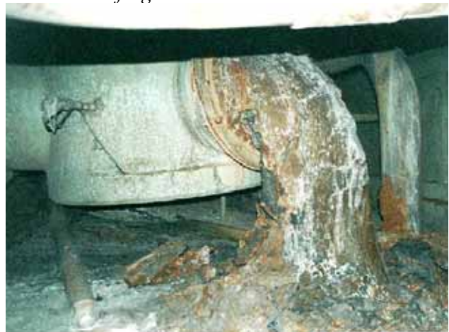
Figure 6 – Lava in steam discharge valve of SDC
