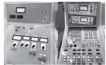
Fig. 2. DT Accelerator Control Panel at KUCA Control Room
