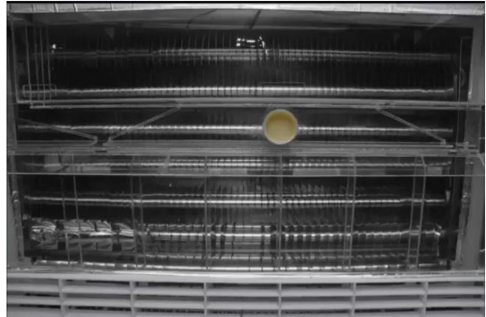
Frost formation on the heat exchanger
