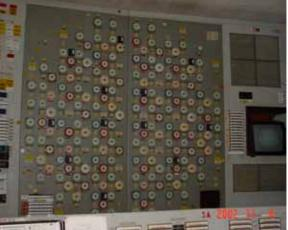
Fig. 11 Control rod position panel of 1st block
