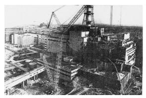
Fig. 7: Construction of Sarcophagus
