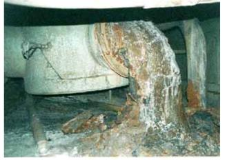
*Figure 6 – Lava in steam discharge valve of SDC*
