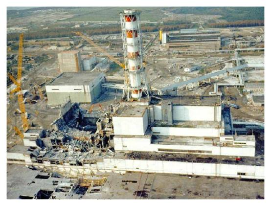
Figure 2 - Destroyed ChNPP Unit 4
