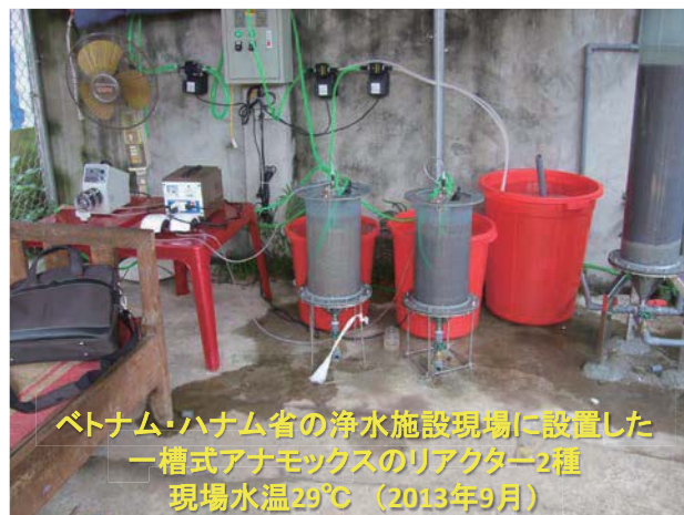
Fig. 7 Small scale one-stage nitrification - anammox reactor installed at the site in HaNam, Vietnam
