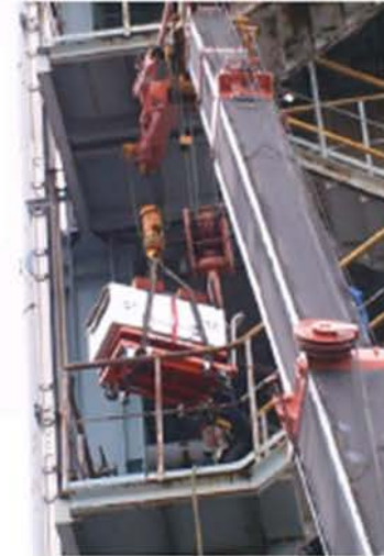
Lifting X-ray Head by crane
